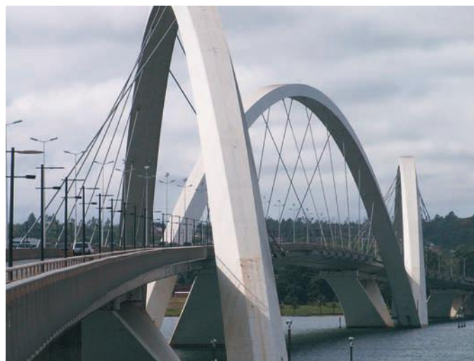
Figure 13.6 This bridge in Brazil uses reinforced concrete.
