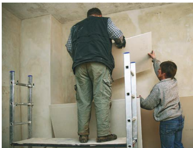
Figure 11.25 This plasterboard is made using calcium sulfate from an FGD plant.
